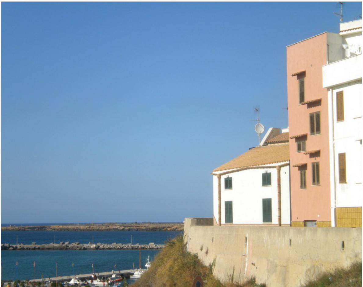
Houses overlooking the sea in Terrasini
